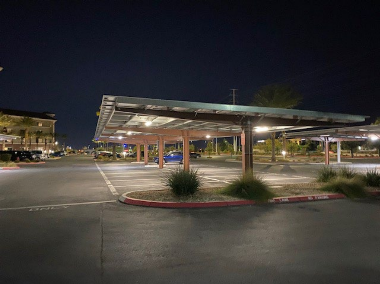
Photo: Example of Parking Lot solar
